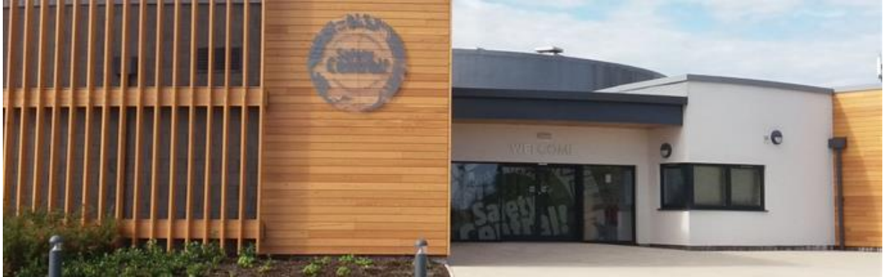
Entrance to Lymm Safety Central
